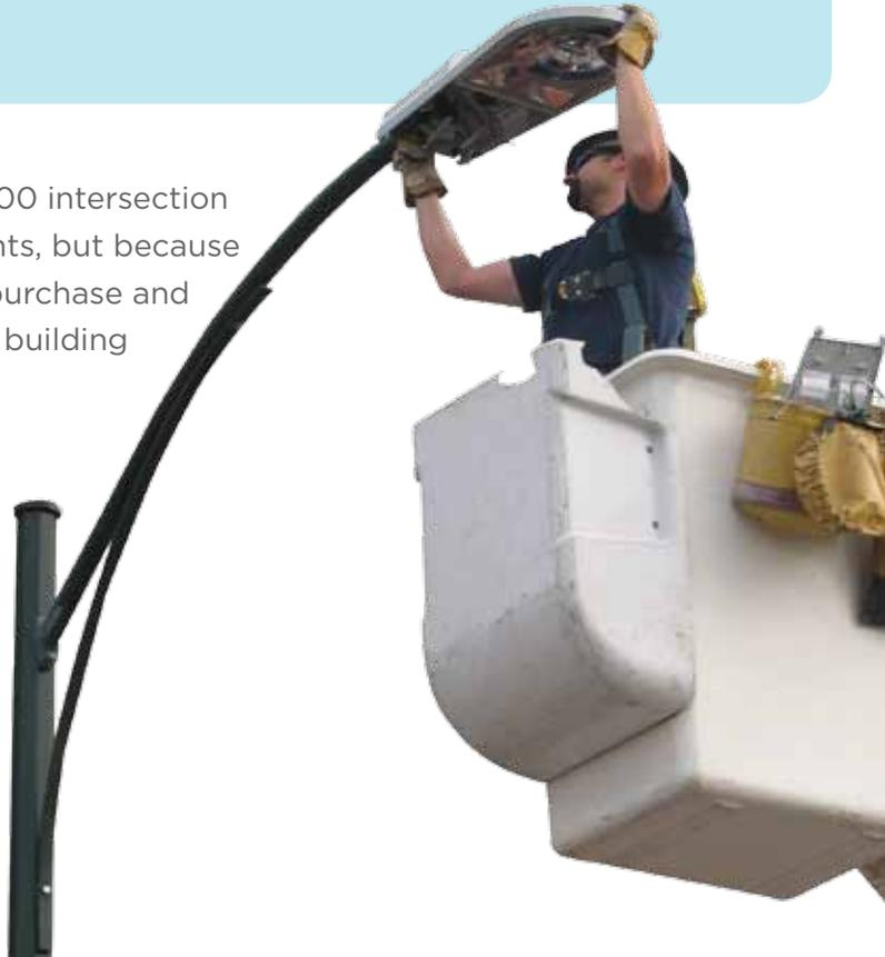
L&P's Brian Zionskowski installs an LED street light in downtown Traverse City. L&P recently completed the installation of over 700 LED street lights, pedestrian lights and building lights.
